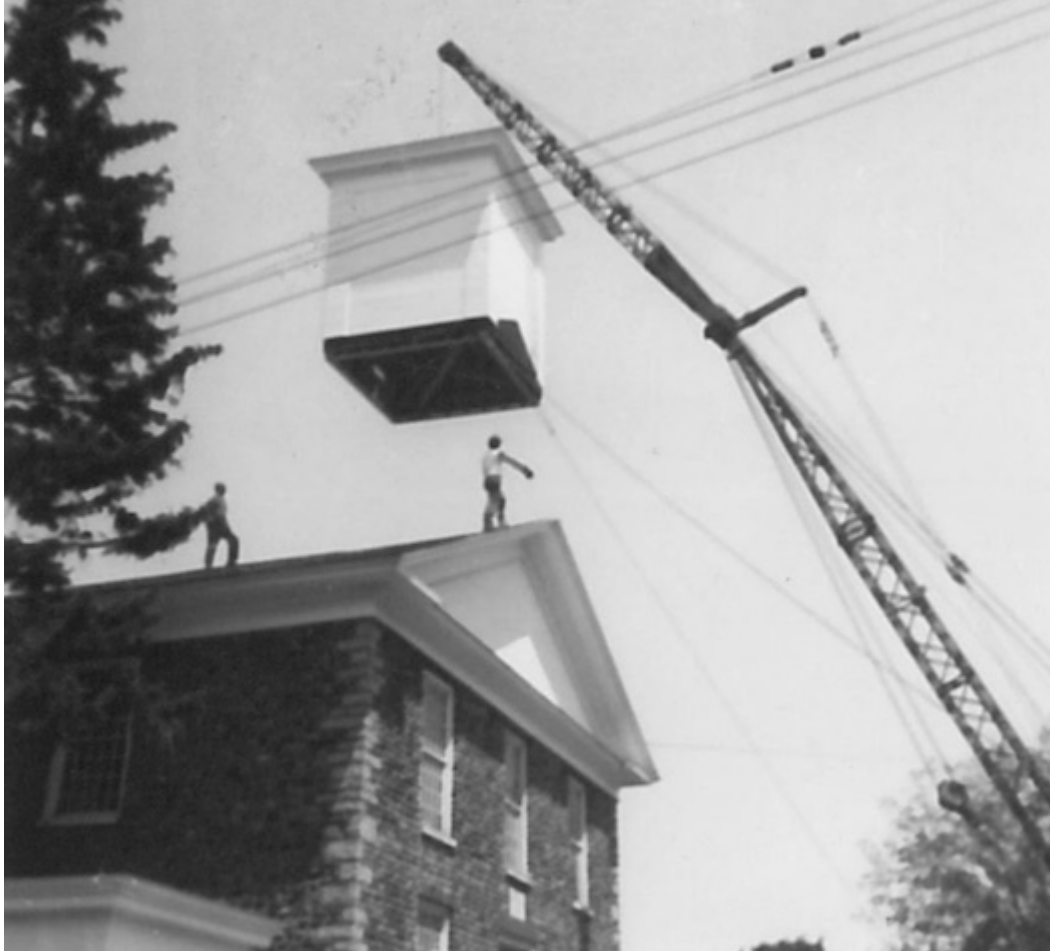
Cobblestone Church tower restoration, 1966
